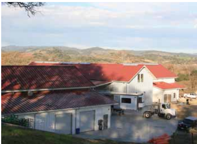
Cary & Associates provided steel and labor for constructing Copain Winery.
