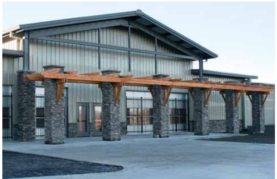
Cary & Associates provided steel and labor for building Kelseyville Lumber.
