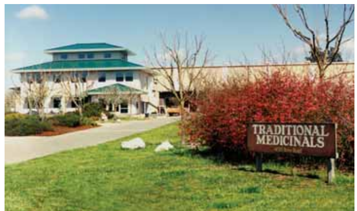
The Traditional Medicinals office complex is one of several buildings Cary & Associates has built for the company.
