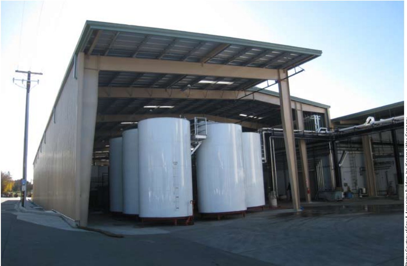
Photos Courtesy of Cary & Associates Builders, Inc./Sonoma Wine Company
